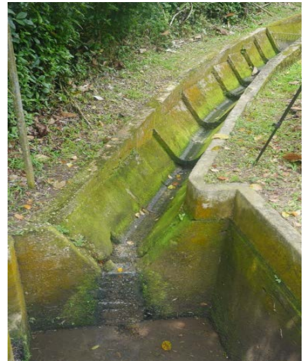
Perimeter Cut-off Drain Within Night Safari
