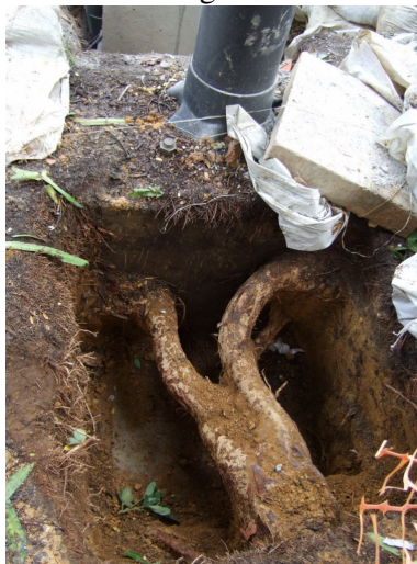
Figure 2: Trial trench by skilled workers using hand tools exposing root architecture
