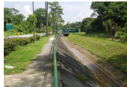
Open air canal along Mandai Lake Road
