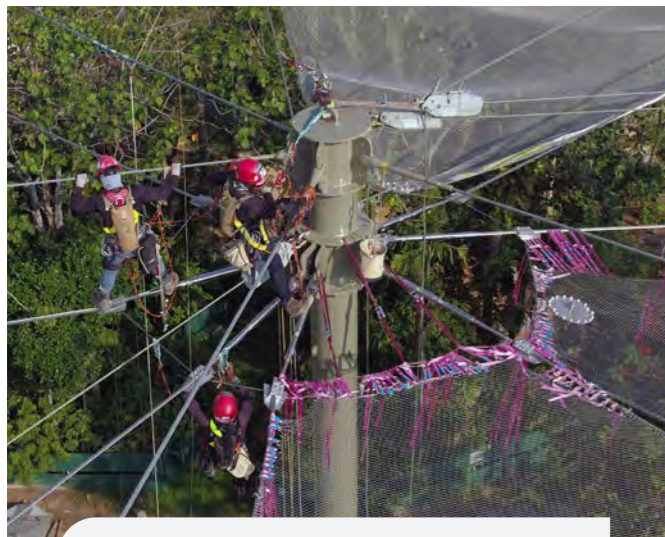
Expert rope accessors take on the tedious and dangerous job of tensioning the pieces of mesh together over the cables.
